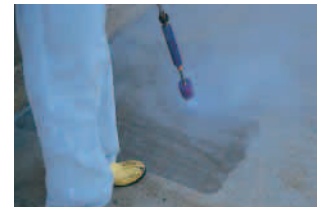
■ Cleaning of concrete surfaces
