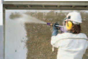
■ Cleaning of facades
