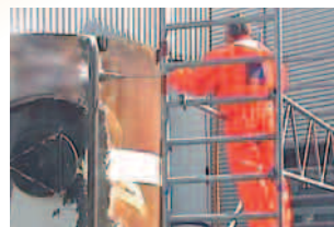
■ Paint stripping, rust removal
