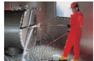
■ Heat exchanger cleaning
