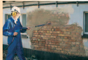
■ Rehabilitation of facades
